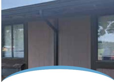
Facia, soffits, gutters and downspouts have all been replaced. The AC covers will also be repaired and/or replaced
