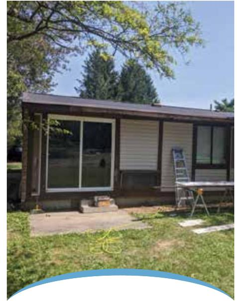
New vinyl siding is being installed over the old plywood panels.
